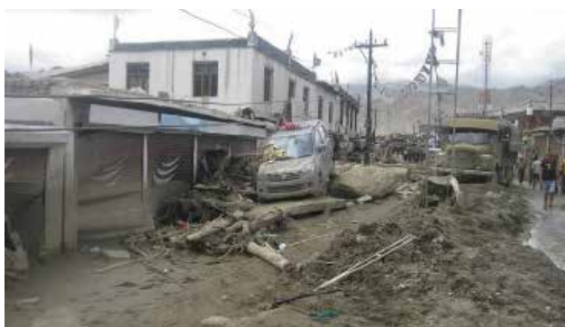
降水や土壌水分が影響する斜面災害 Landslides at the slopes triggered by heavy precipitation and/or wet soil conditions
